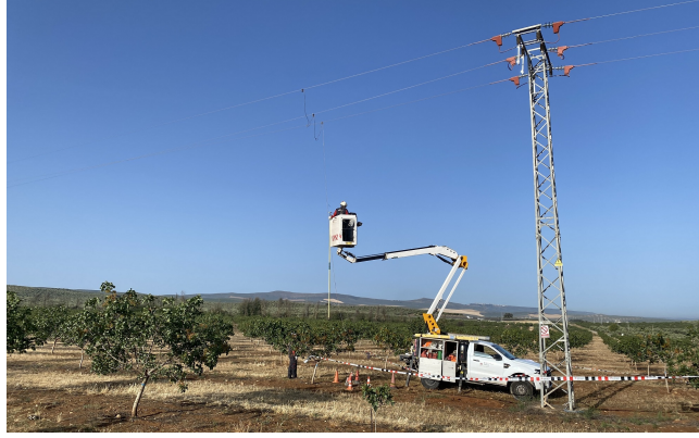
Figure 1: Human operator on elevated working platform grounding the three phases of a power line section close to the ATLAS Flight Center before conducting a maintenance task.
